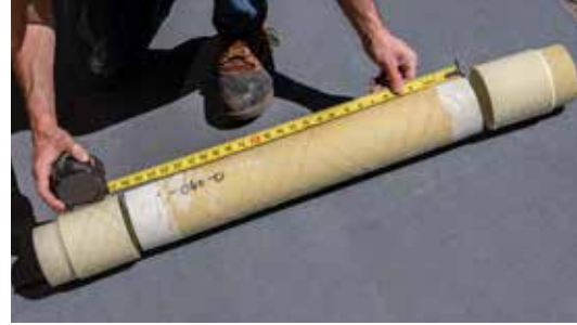
3. Verify overall length of assembly by dry-fitting on tank top. Prep joint surfaces.
