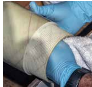
6. Check ID of joint for adhesive overflow, wipe away excess.
