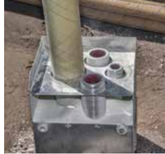
2. Taper riser pipe. Verify taper and re-taper if necessary (see Average Taper Dry-Insertion Length table).
