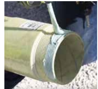
7. Apply thread dope to adapter threads.
