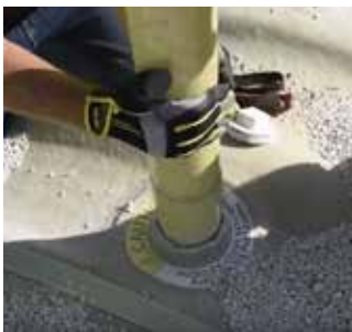
8. Thread Riser Pipe assembly into tank top fitting.
