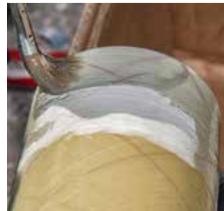
5. Apply thin layer of adhesive (see Adhesive Kits table).
